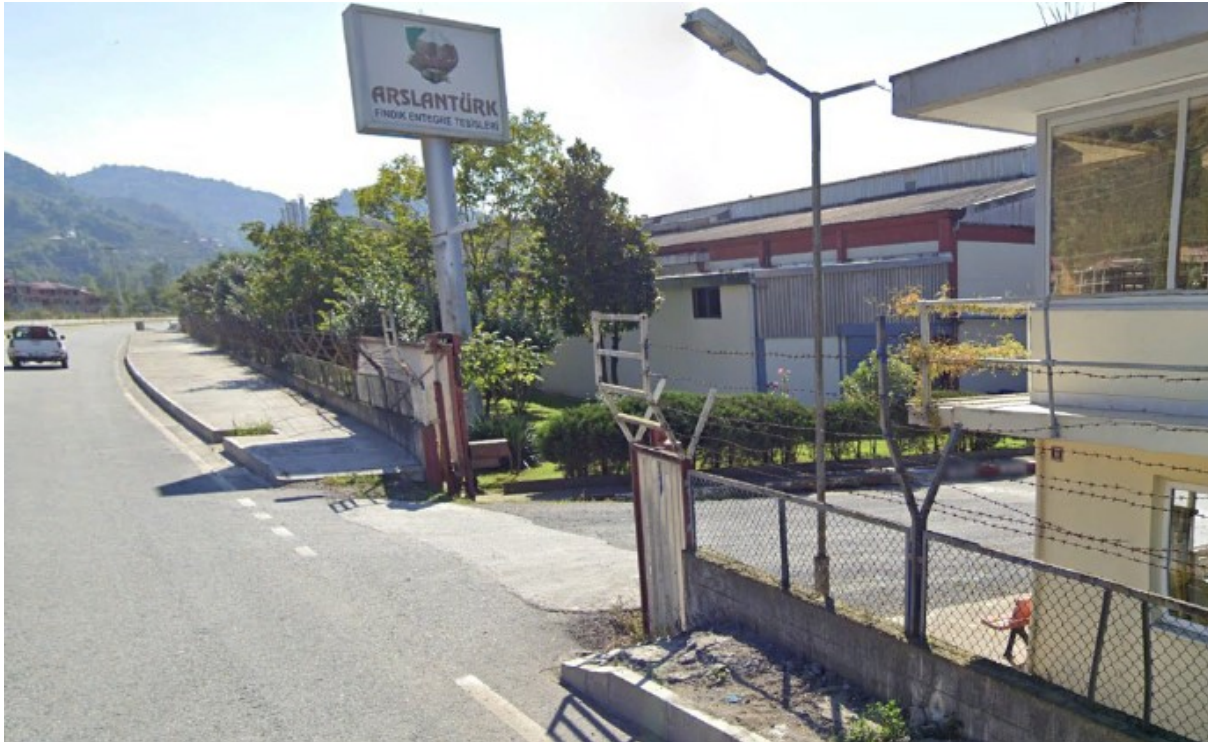
Street view entrance to the Arslanturk factory 23
