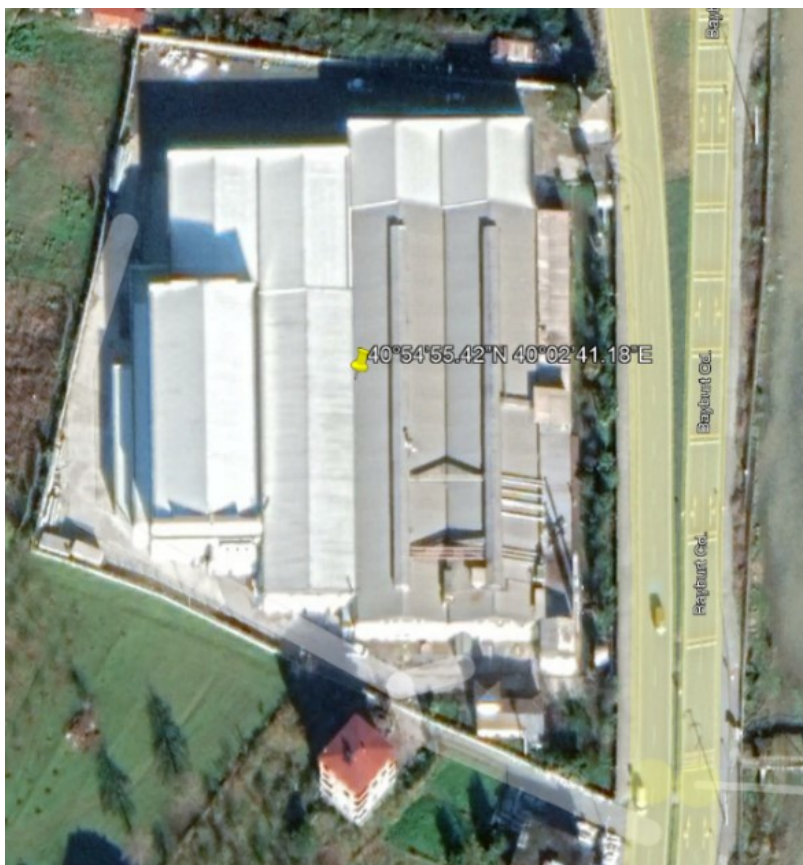
Aerial view of the Arslanturk factory 24
